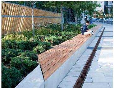
Seating integrated into retaining wall<sup>4</sup>
