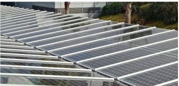
hotovoltaic solar shading structure to car park.7
